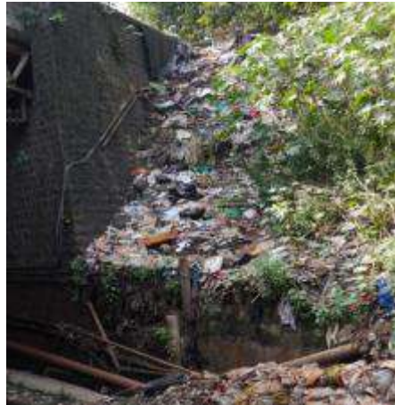
Along railway tracks and other leakage points
